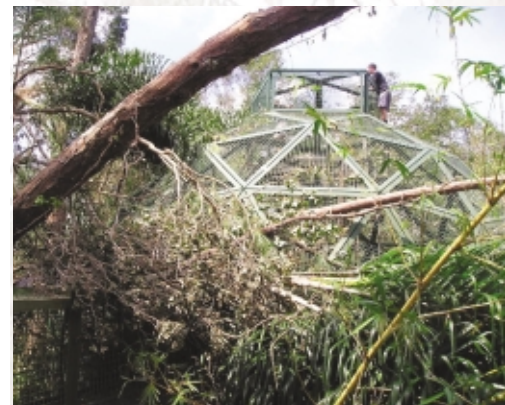
Fallen trees surround the Orang dome after Hurricane Charley
